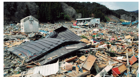
Tertimbun puing-puing akibat tsunami besar (Kamaishi, Iwate. 4 April 2011. Sumber: Kochi Post)
